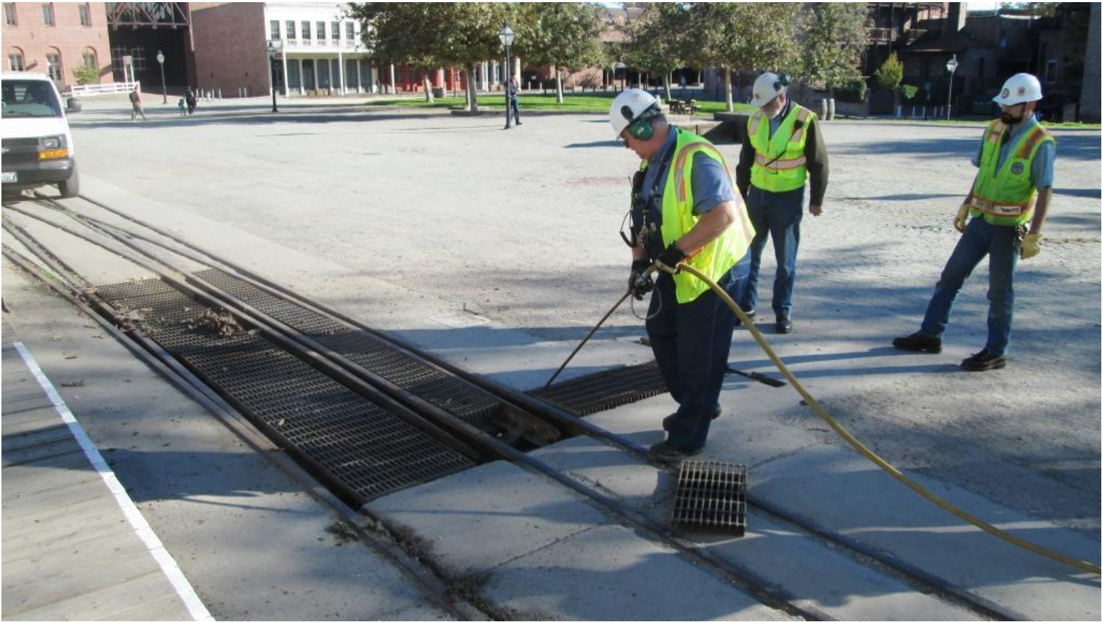
Chris uses the air-wand to blow debris out of the dual-gauge switch
