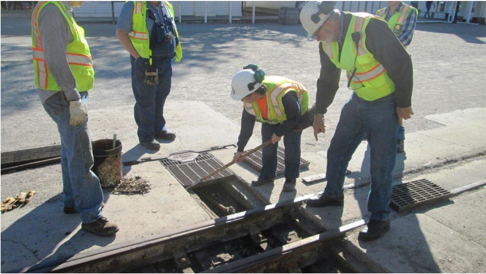
Pam cleans-off the area supporting the grate over the switch-rod
