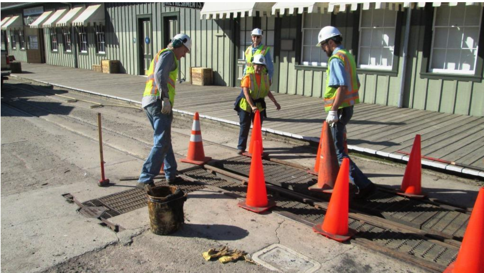
Pam, Steve, and Matt B. put safety cones around the switch to alert folks to the potential trip hazard
