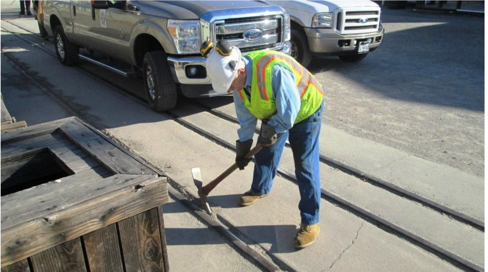
Clem digs the dirt out of the flange-ways on the dual-gauge Display Track
