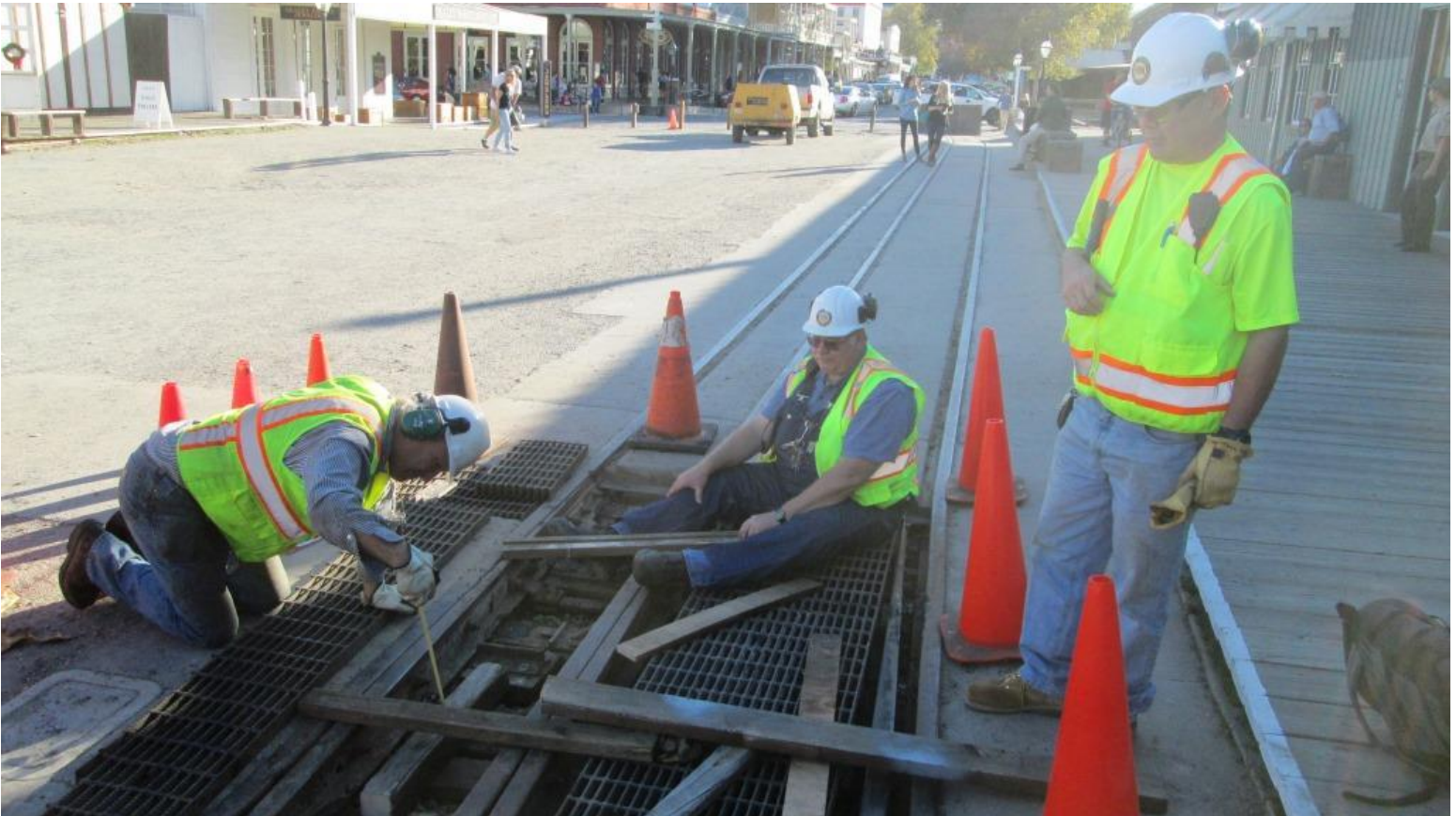
Steve, Chris, and Taka build a new support system to hold the grates in place
