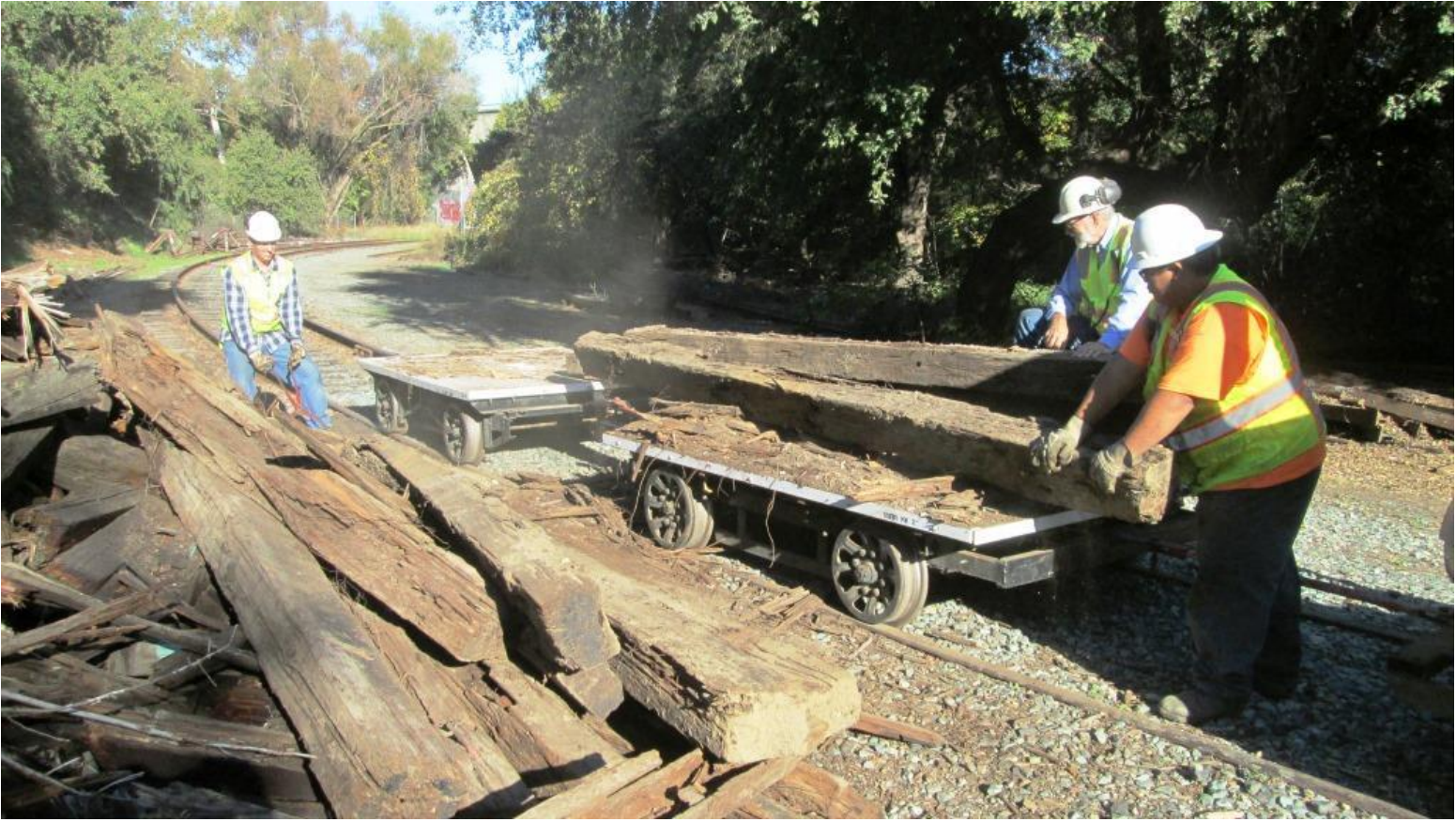
At Setzer, Alan supervises Weston and Anthony as they make "Mount Dead Tie" grow...
