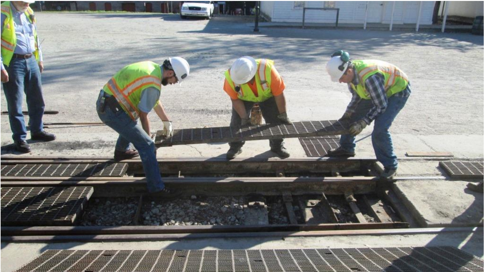
Matt B., Anthony, and Weston temporarily replace the unsupported grates over the switch
