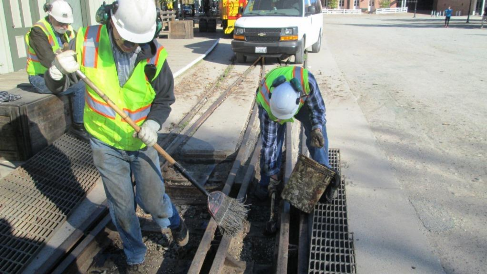
Steve sweeps the dirt and debris off the switch-plates to which Weston applies grease
